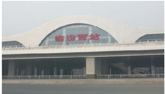
Shanxi Linfen High Speed Rail Station
