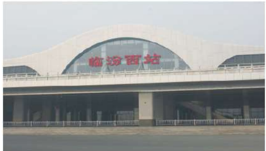
Shanxi Linfen High Speed Rail Station
