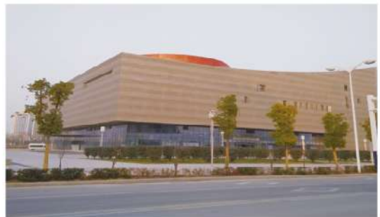
Shanxi Tongmei Group Zhangze Power Puzhou Power Generation Branch
