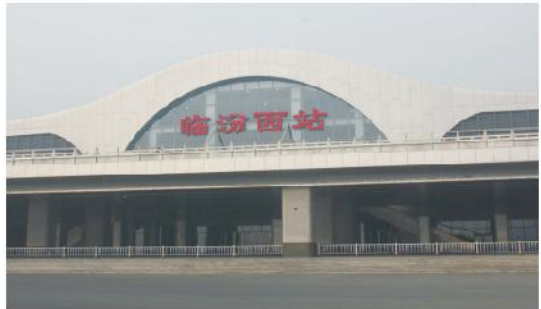
Shanxi Linfen High Speed Rail Station
